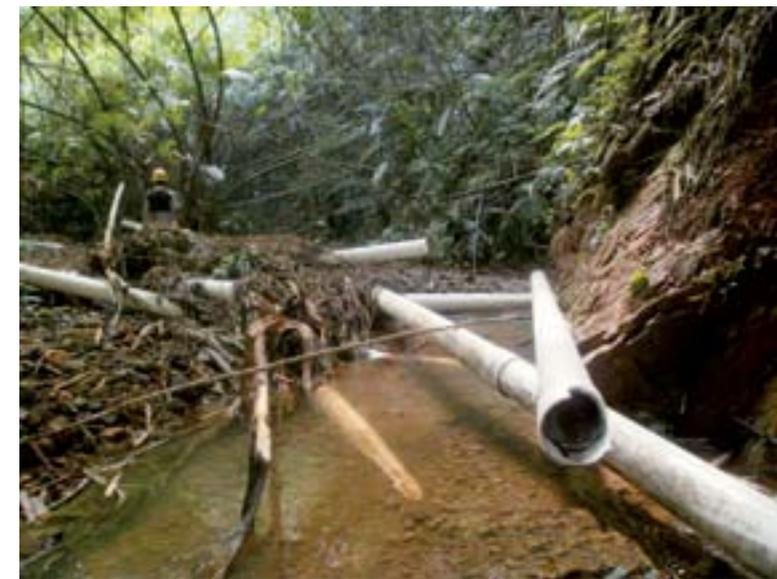
Photo: Water supply pipe washed away by stream flood in Maliyang relocation camp on September 19, 2012.
